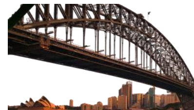
Bridge Lifting and Installation, Large-scale Structural Movement Platforms
